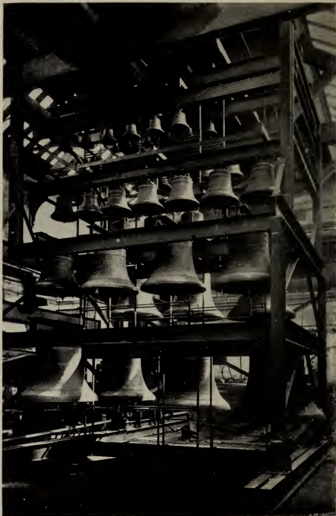
LOUGHBOROUGH: THE CARILLON FRAME MODERN CONSTRUCTION
